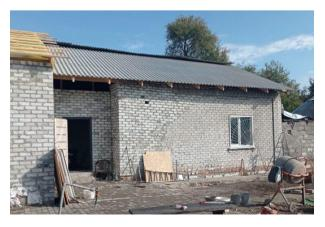
Consequences of shelling. Holes in the walls of the house are repaired
