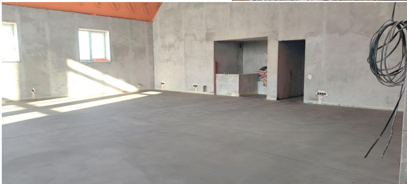
Our auditorium is prepped to be overlayed with tile.
