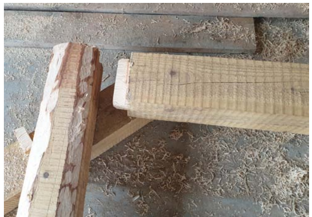
Tongue & groove with a chainsaw and tape measure!
