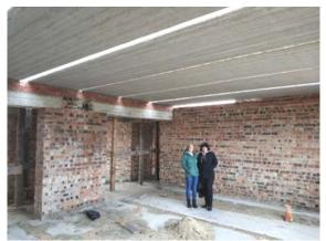
Sveta & Marina stand alongside a wall in building! The slabs have been set above and you can see the cracks between the slabs. These are the cracks that need to be filled in so there will be a solid covering.
