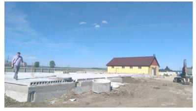
because they had to lay foundation in deeper in some areas where they had to dig more to get to good and firm soil. It is as deep as 2.7 meters in those areas instead of 1.2 meters planned. It is due to the bad soil. Since there used to be a landfill there, 60% of the foundation is 2 to 2.7 meters deep. This situation was explained to you as you visited the construction site. But now all of foundation is on solid ground.
