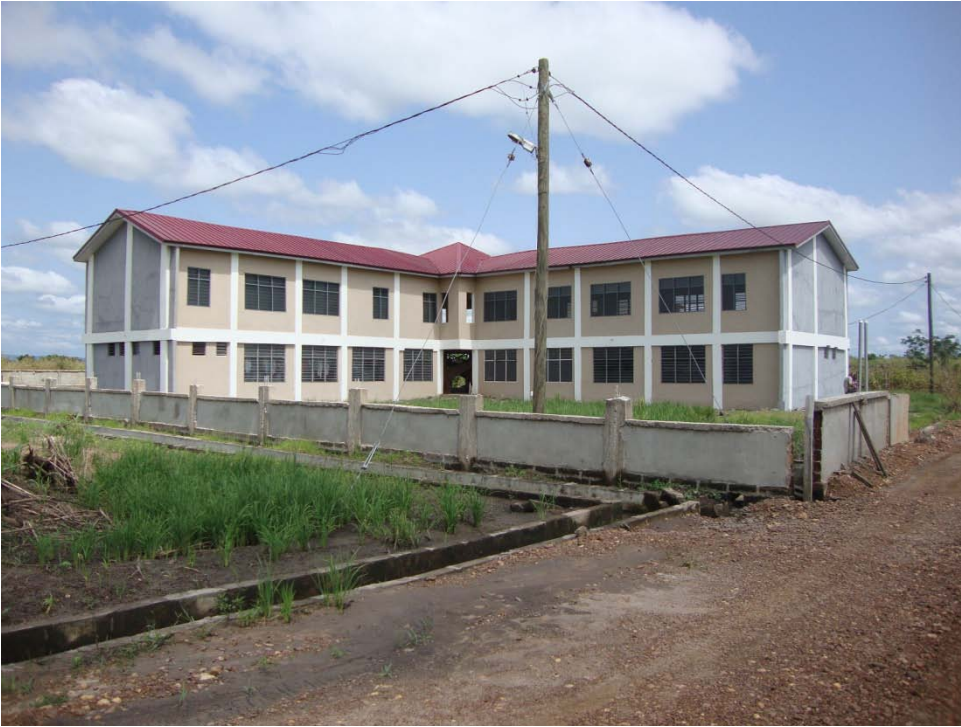
Newly constructed facility – Volta Bible College
